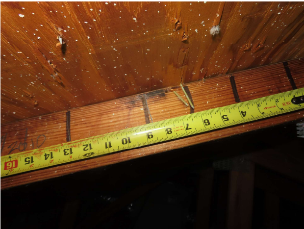
Roof deck nail spacing - Edge
