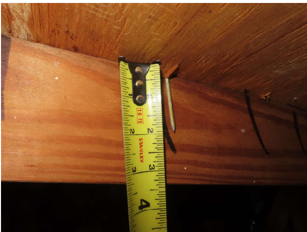
Roof deck attachment - 8d nails
