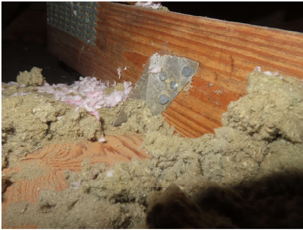
Roof to wall attachment - Clips
