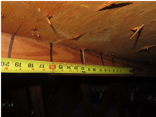
Roof deck nail spacing - Field
